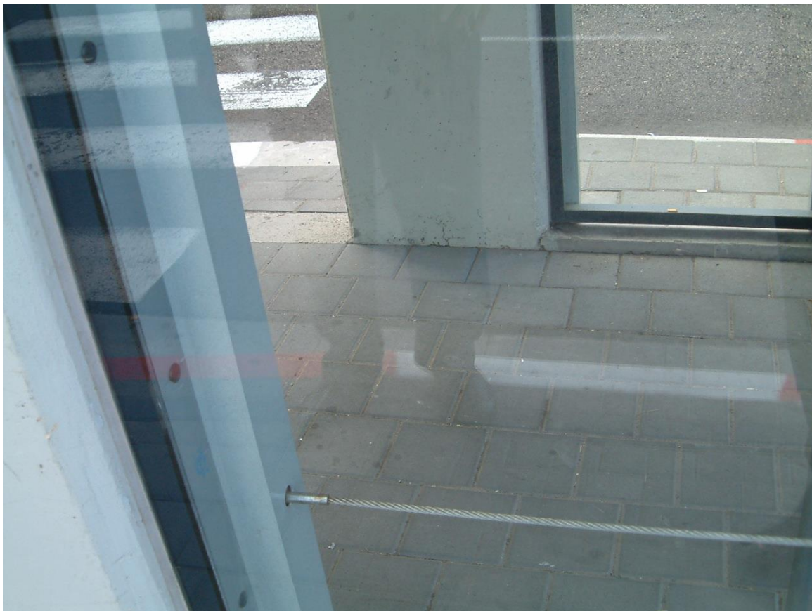
Laminate glass with blast energy absorption
