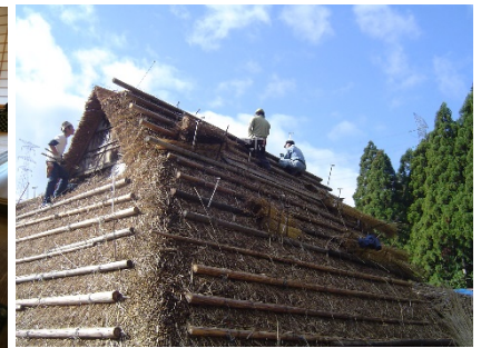
Thatchers working on the roof
